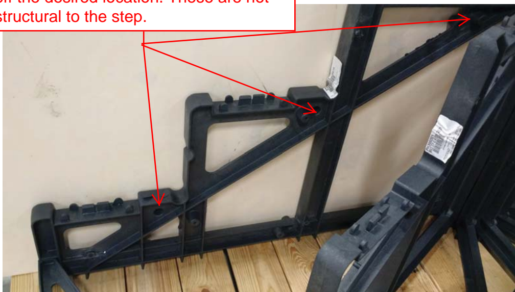
Installing the screws can make it difficult to fit the shell on the step.
